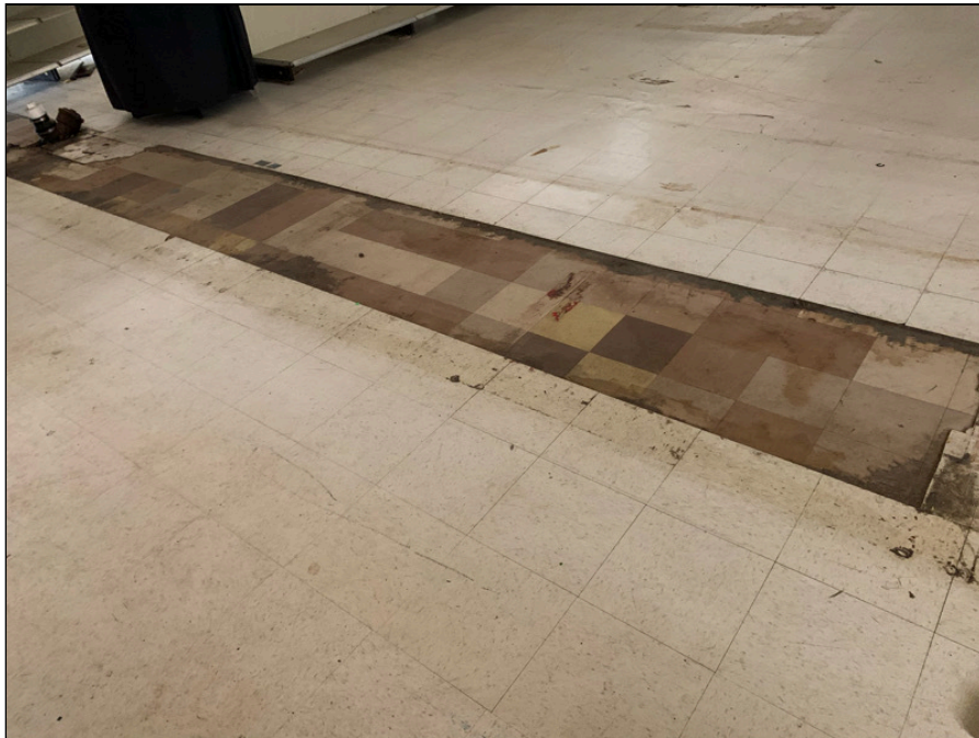
2 - 9x9 floor tile located below 12x12 floor tile throughout the store with positive black mastic
