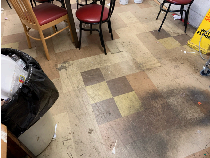
1 - Asbestos containing 9x9 inch floor tile and associated black mastic
