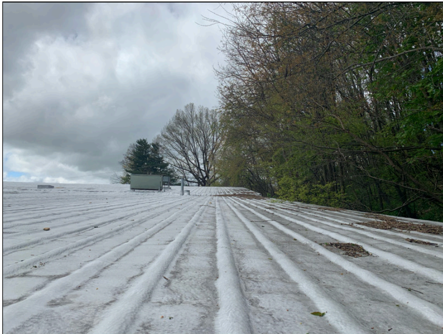
4 - Roof - silver paint located on metal roof below foam
