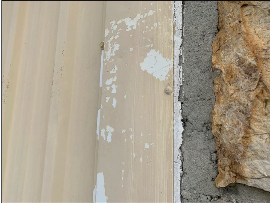
3 - Asbestos containing white (hard) sealant along exterior walls
